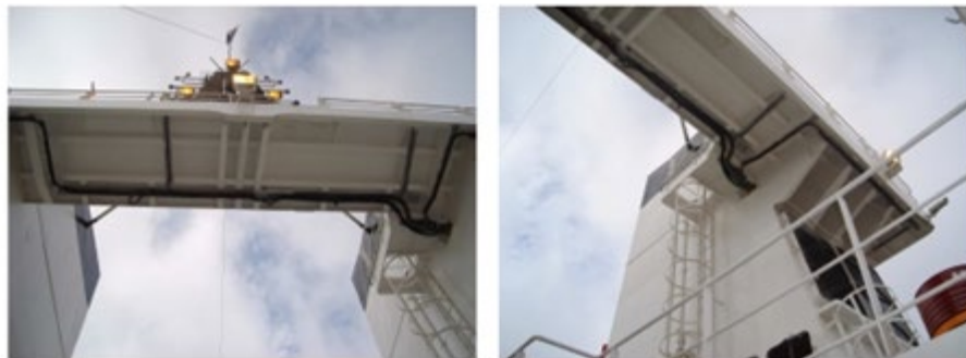
Typical Cable installation in Bridge Mast Area
