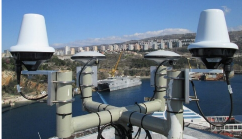
Drip loops and spare coils
