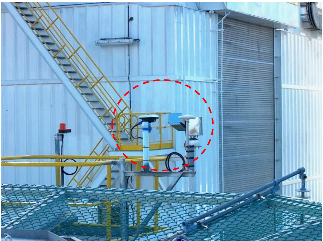
Antenna installed on main deck level underneath derrick base structure; signal masking and multipath experienced
