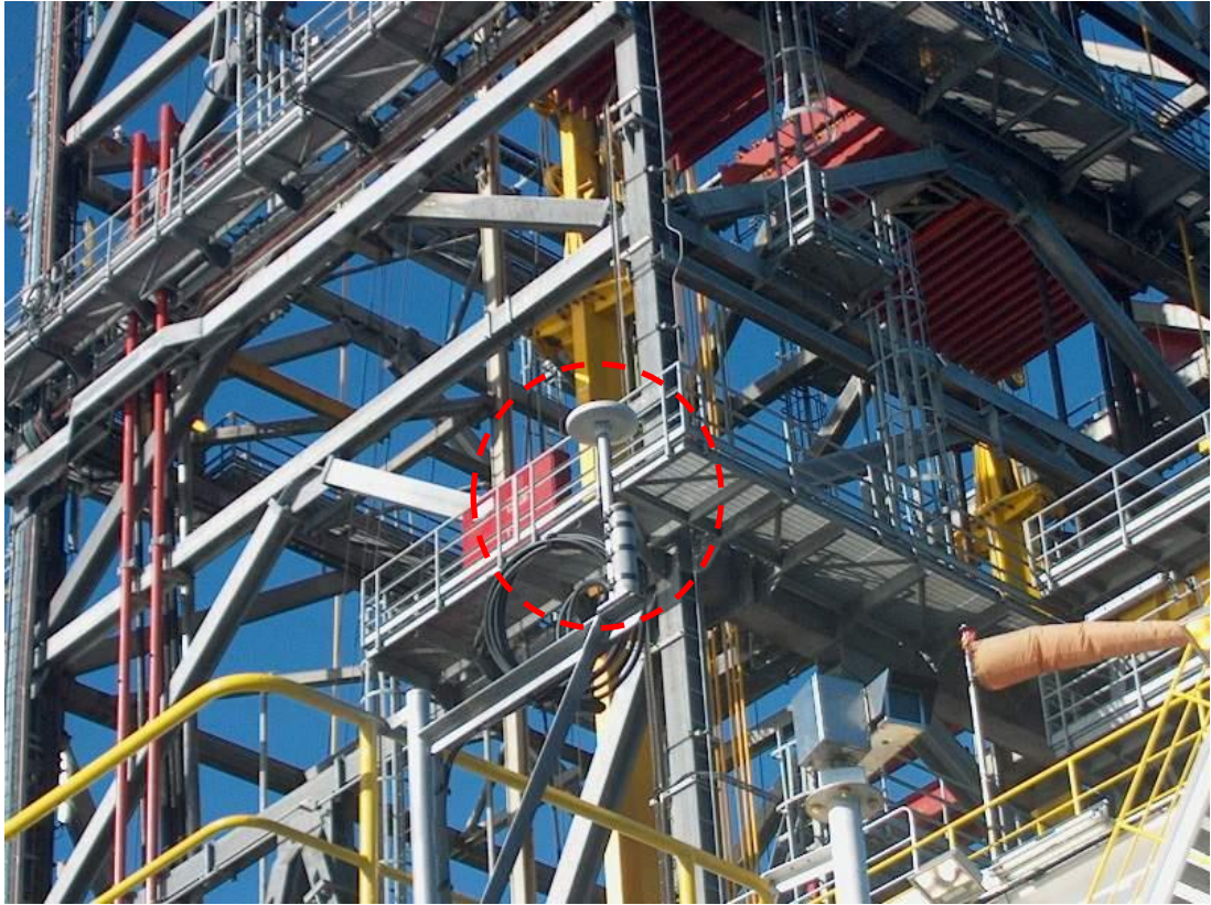
Antenna installed on main deck level underneath derrick; signal masking and multipath experienced
