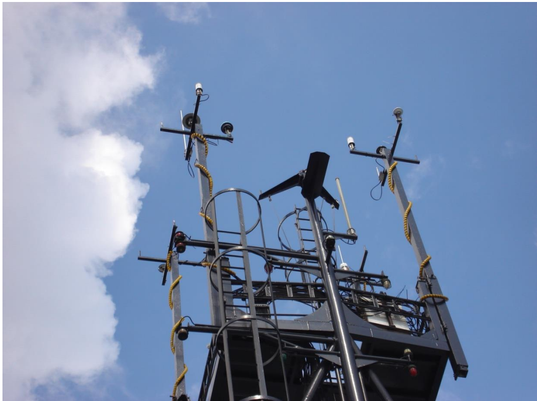
Antennas installed at top of mast on retractable mast extensions with good spacing.
