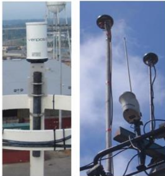
Figure 13. Examples Antenna Fixing Arrangements
