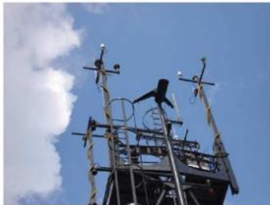
Fig 11. Good Installation – Antennas Installed at top of Mast on Retractable Mast Extensions with Good Spacing.
