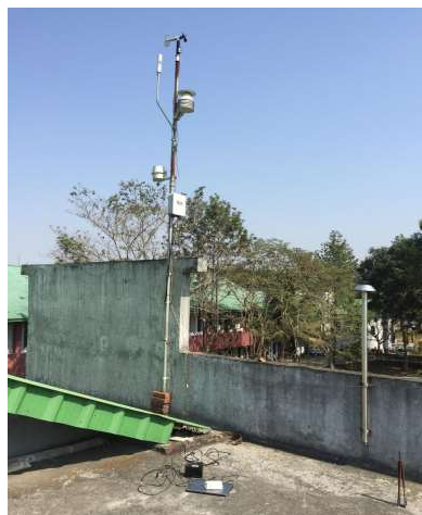
Figure 14: Photo of the weather station causing the interference in the India case study
