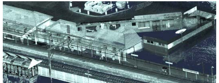
Stencil captured fine details such as overhead wires at this light rail station. The scan's 72,000,000 points of data were captured in the 20 minute interim time between trains.
